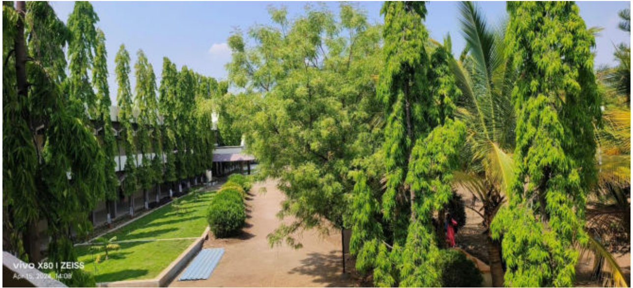
College main building
